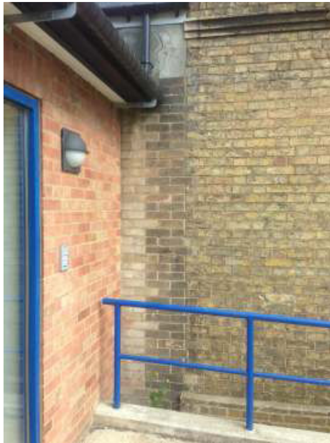
Detail of the toothed-in brickwork to west of original house showing three phases of change during the 1950s and 1960s to the original Victorian building
