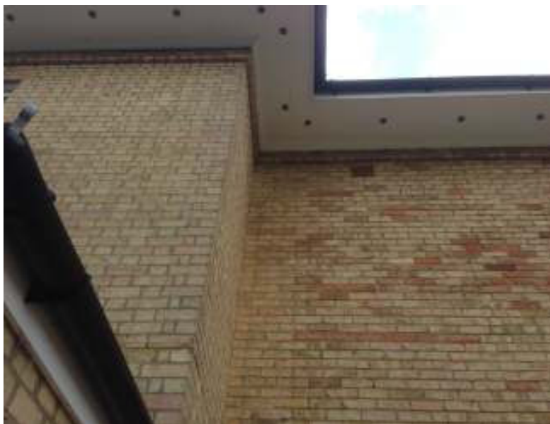
Original Villa with simple over-sailing courses copied on the modern stretcher bond, cavity wall extension using reclaimed bricks and four-board copy of the original soffit
