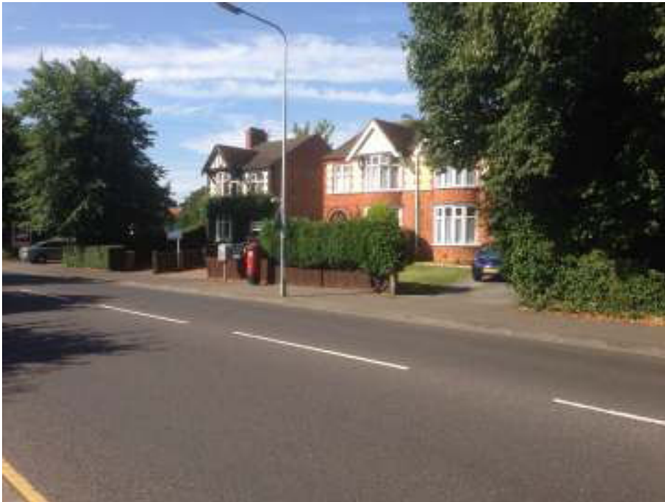
South view from the east side of Eastfield Road showing how the subsequent development to the north effectively screens the building from view
